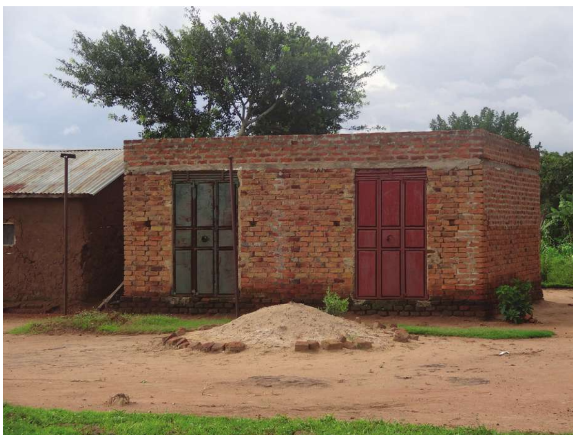
Plate 4 : Rooftop blown off by strong winds in Bulange sub county
